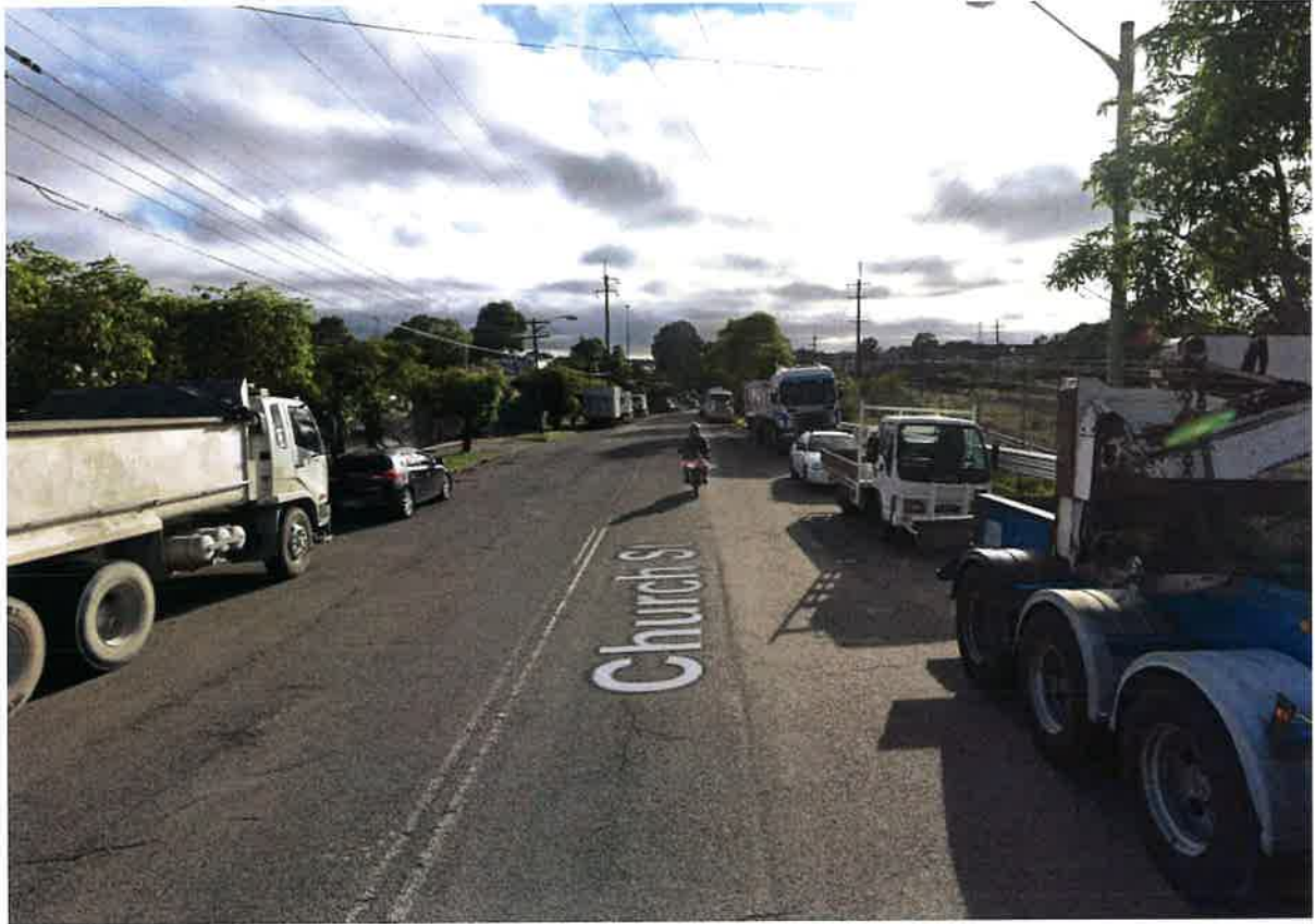
Figure 2 – Church Street local road
