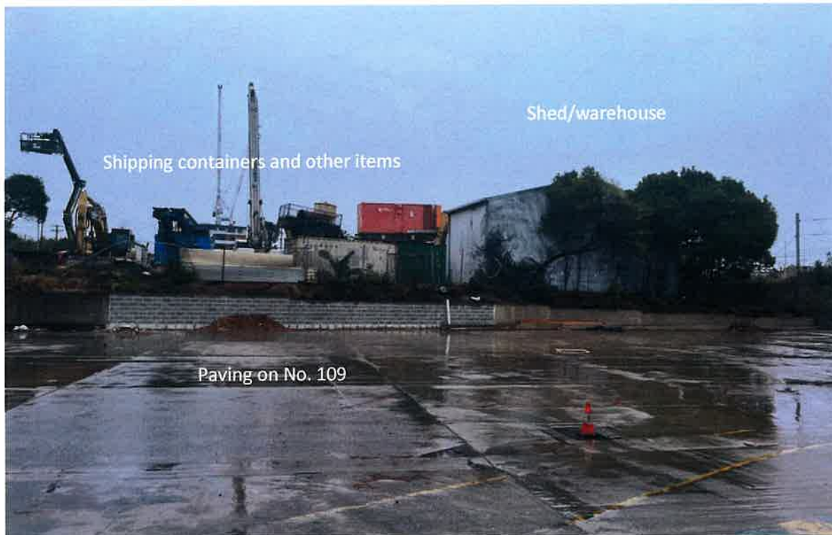
Figure 2 – Development site viewed from 109 Church Street (from the east)
